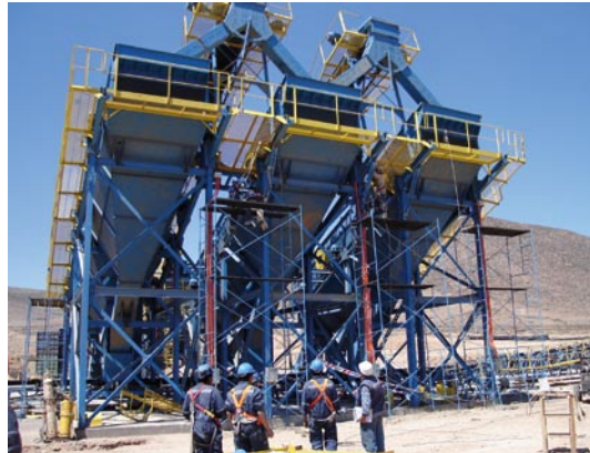
Conveyors from crushers being connected to high speed drums and hoppers.
