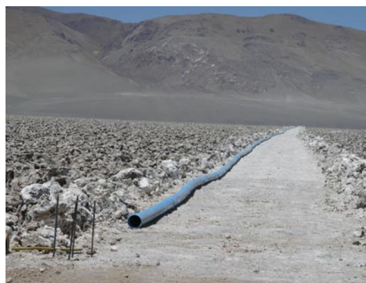
Production pipeline being laid for pumping brine to evaporation ponds.
