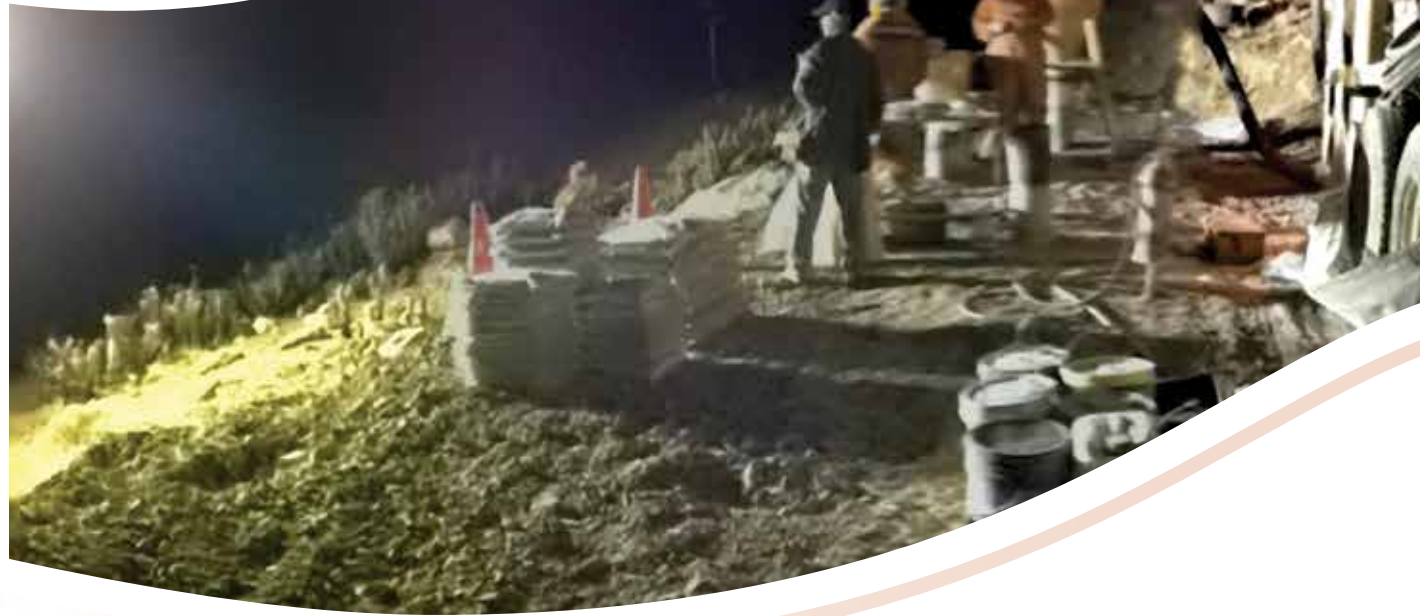
Night shift drilling at Soberana (July 2012)
