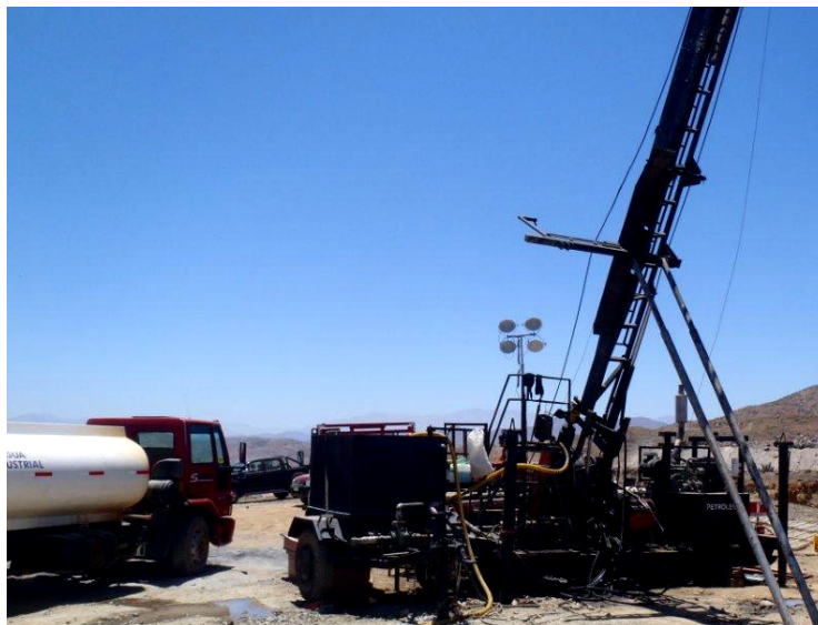
Diamond drill rig set up at AD-05 platform at Mariposa.
