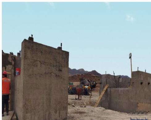
Foundation for the Two Ball Mill Machines
