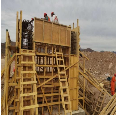
Foundations for the Crushing Machines
